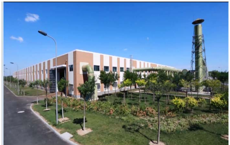
Tianjin Compost Facility and Biofilter Discharge Stack
