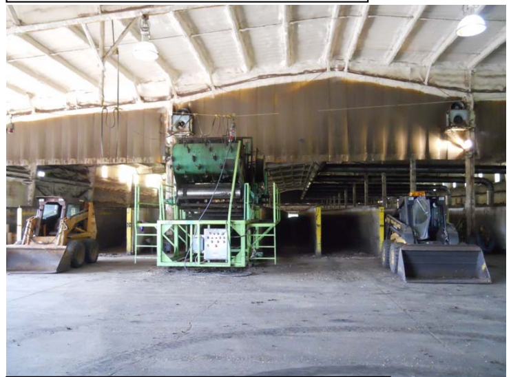
Loading Area with Stayflex Coating
