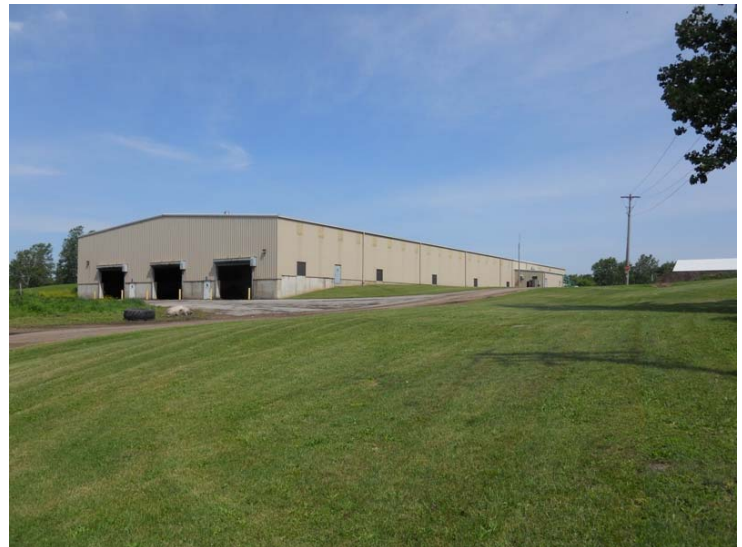
Lockport Facility Showing Discharge Pit Design
