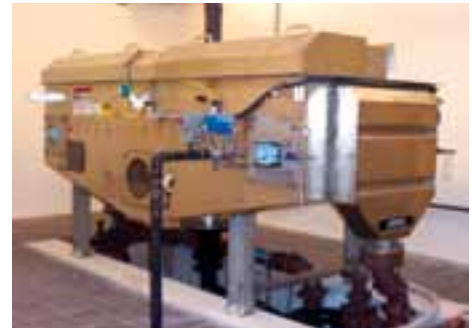
Rotary Drum Thickener
