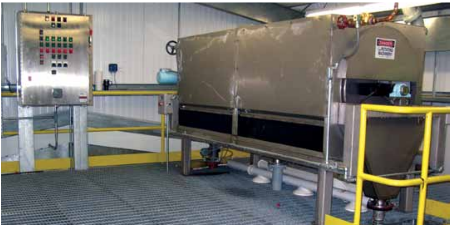
Filtrate Drips into Stainless Steel Drip Pan
